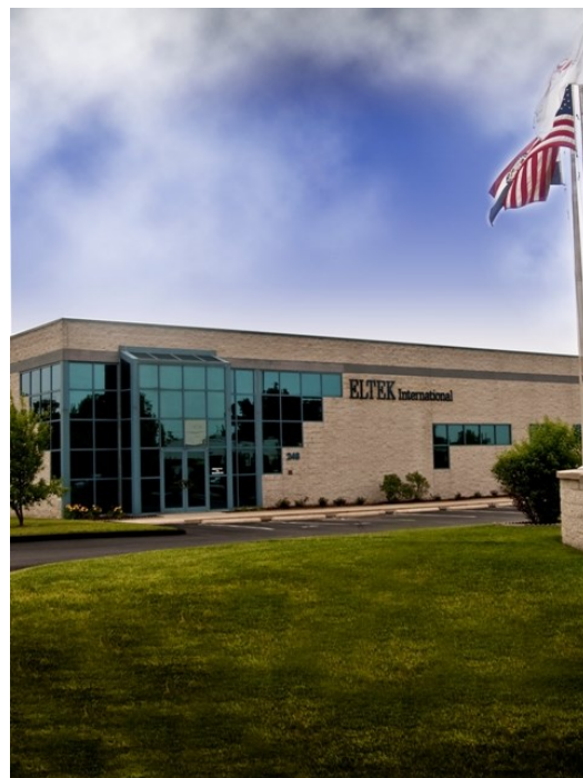
ELTEK Labs facility in St. Charles, MO, U.S.A.
