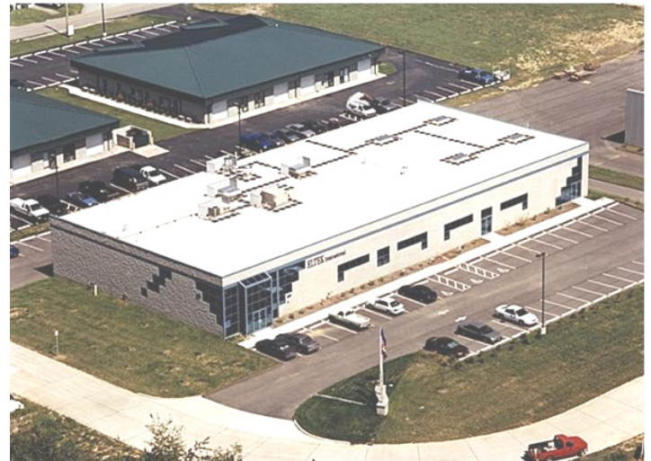
ELTEK's headquarters in St. Charles, MO, U.S.A.
